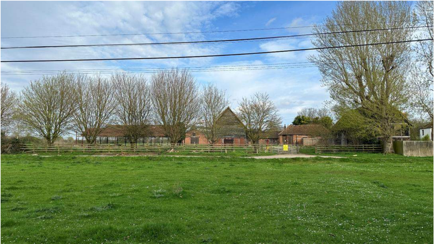
Current view of Site
