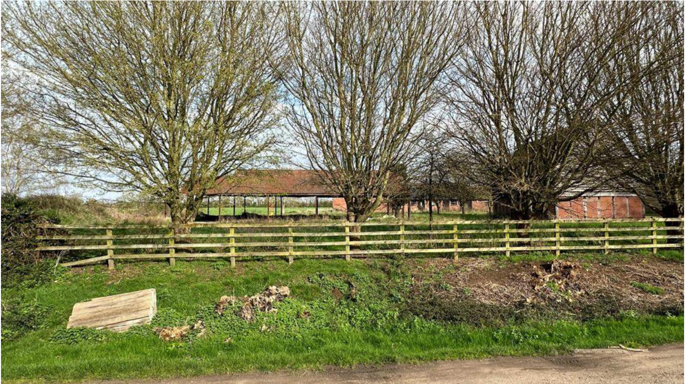
Current view of Site (showing open barn – to be demolished)
